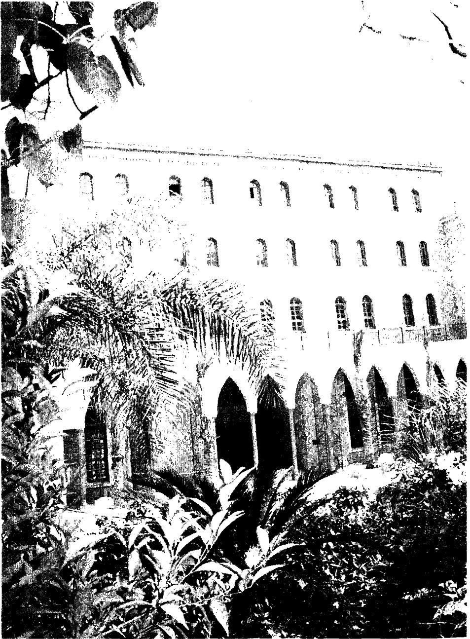
The newly completed College Hall
