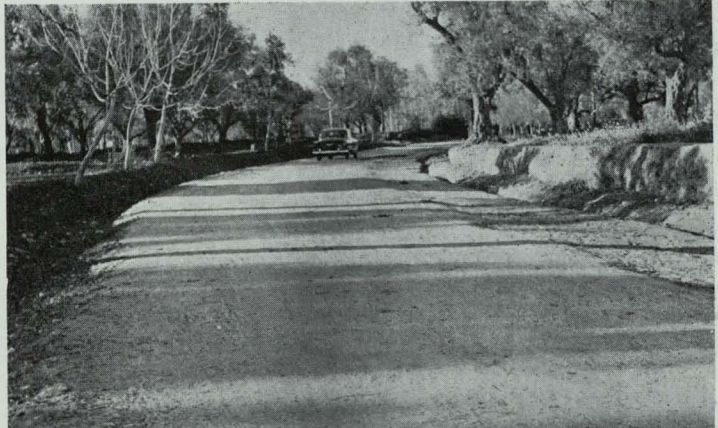
Diatol Roadway at Harrasta, Damascus Syria. Const. July 1954. Left unsurfaced, by P.W.D. Order
