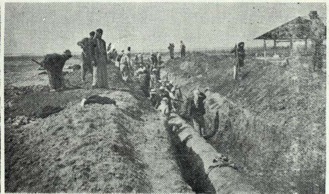
Wrapped pipe in Ditch and Filling
